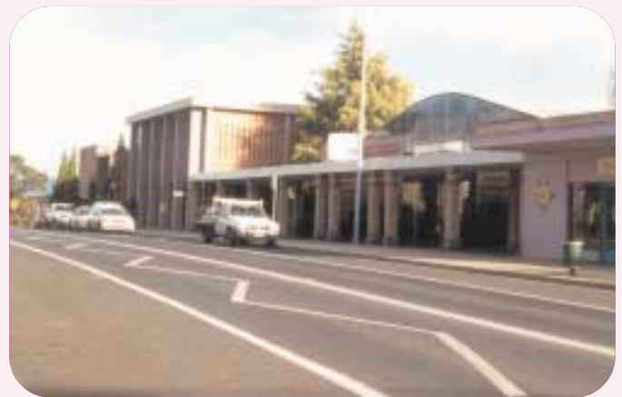
Mort Street, the main thoroughfare through the centre of Lithgow showing (from the right of the picture) the Business Enterprise Centre, the Centrelink office and Lithgow City Council Chambers.
